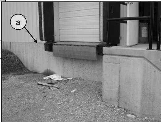
Slab-on-Stem-Wall-with-Fill, Without Attached Garage
