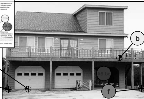
Elevated on Piers, Attached Garage, Partial Obstruction
