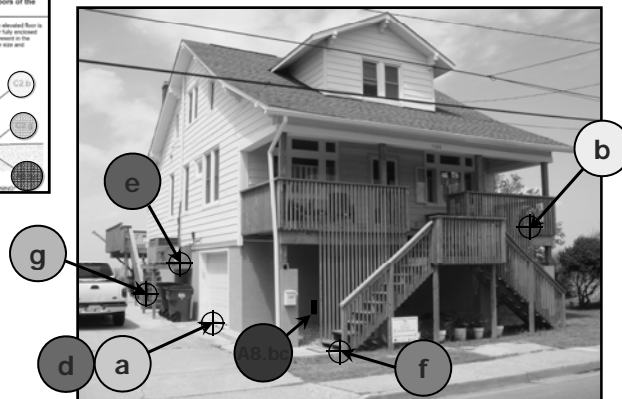
Full Story Basement Foundation, Fully Enclosed, Used as the Garage
