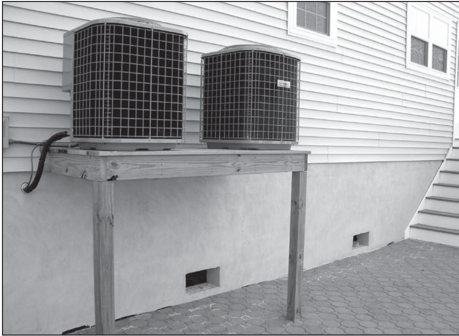
Figure 19. Foundation wall with omitted blocks as flood openings (insect screen not visible)
